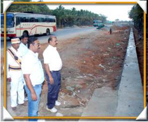
Fig: Inner Ring Road – Renovation work
