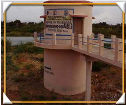
Fig: Intake well
