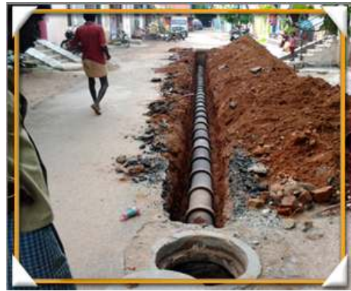
Fig: Pipe Laying – Under Ground Drainage
