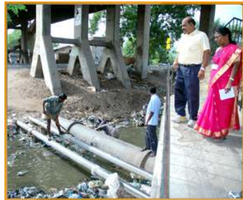
Fig: Desilting of Channels
