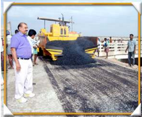
Fig: Commissioner visit – Road Work
