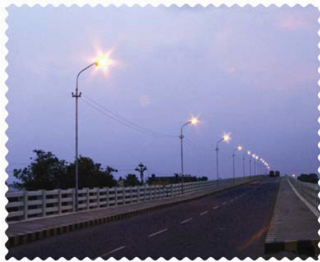
FIG: Street Light in Bridge
