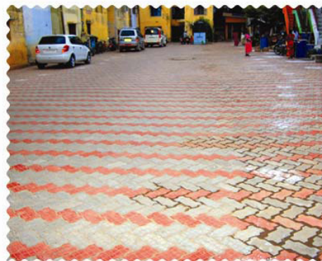
FIG: Paver Block Road – K.K. Nagar
