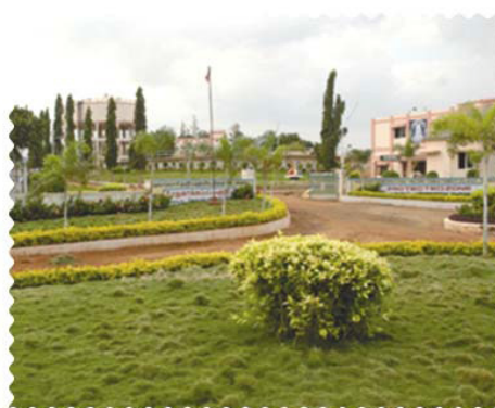
FIG: Vaigai Water Supply II Phase
