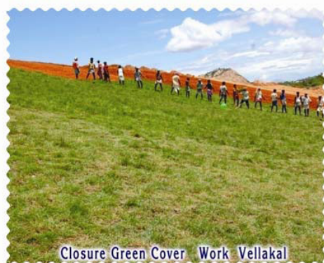
FIG: Closure Green Cover Work Vellakal
