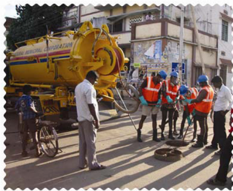
FIG: Scavenging Lorry
