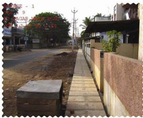
FIG: Road Side Storm Water Drain
