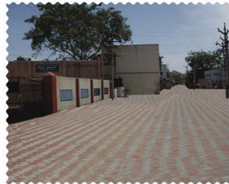
FIG: Paver Block Road
