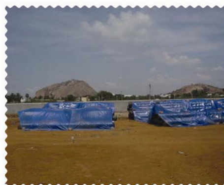
FIG: Closure Green Cover Work Vellakal
