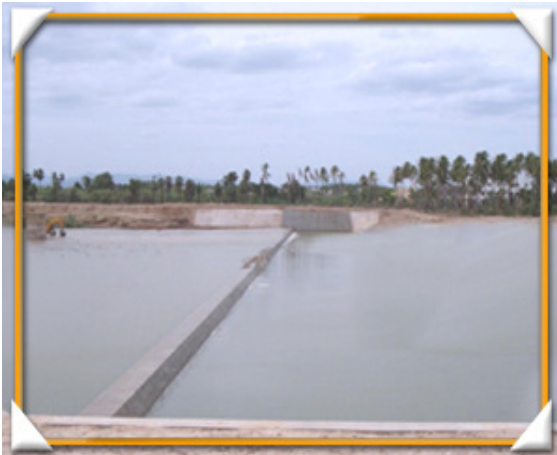
Fig: Check Dam - Manaloor
