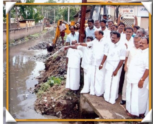
Fig: Desilting of Channels
