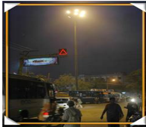
Fig: High Mast – Anna Nagar Junction
