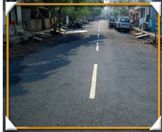
Fig: Renovated road – Anna Nagar
