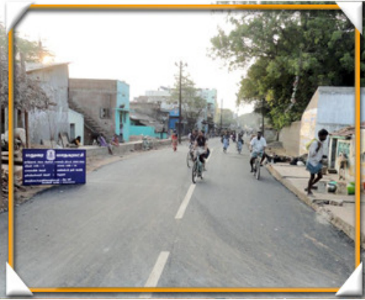
Fig: Renovated road - Munichalai
